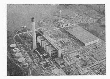
The 2,000 megawatt oil-fired power station at Pembroke is at present under construction. Already two of its four 500 megawatt turbo-generators are in partial service. The third should be in use by May, 1971, and the fourth by January, 1972.
